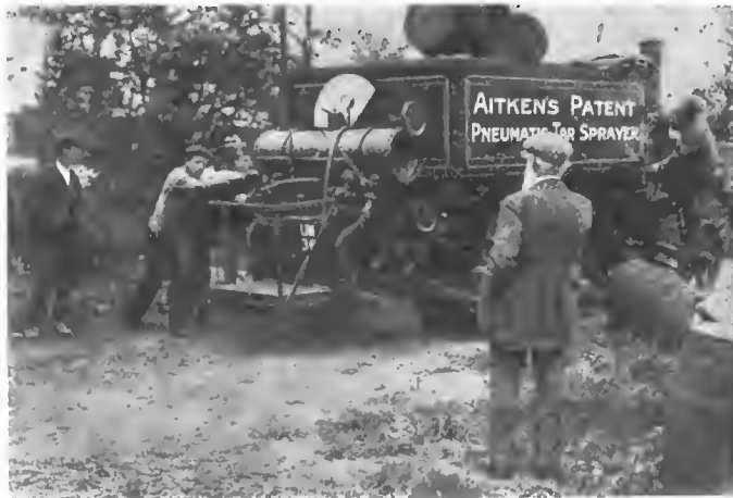
A TAR SPRAYER AT WORK ON THE ENGLISH ROADWAYS.
